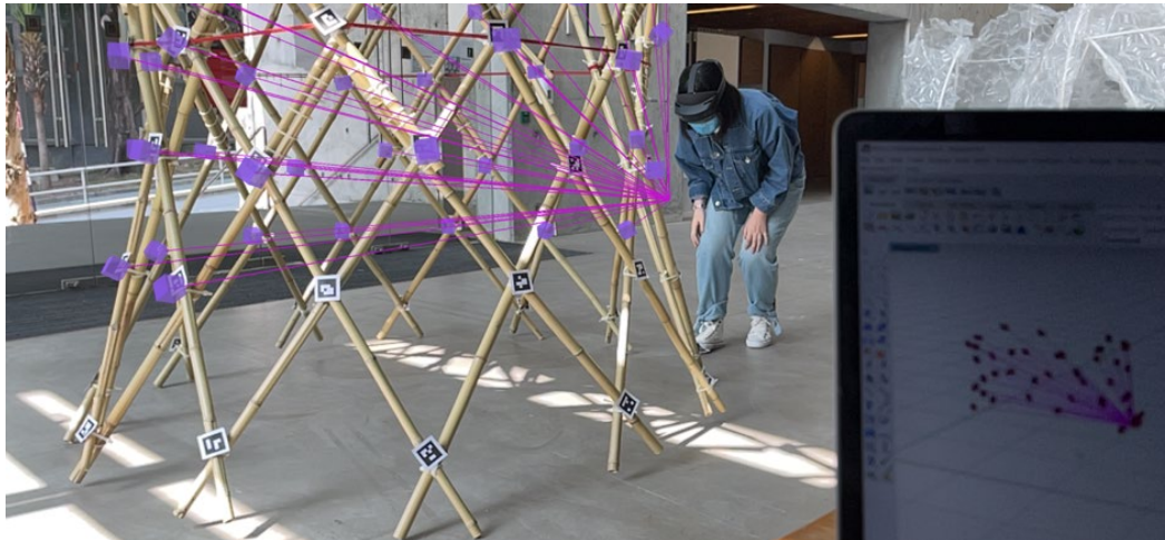
Figure 14. Scanning Aruco markers on the installation. Live stream between Rhino and the HMD to bring the tracked points back into a 3D environment.
