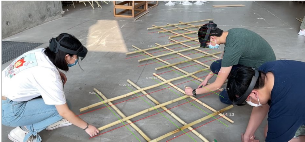
Figure 12. Grid layout and marking through holographic guidelines.
